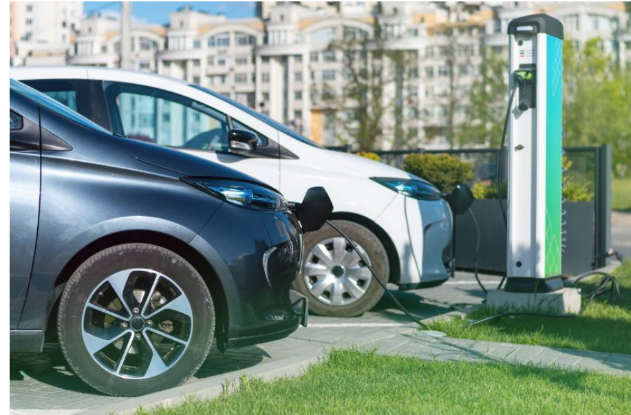
Electric Vehicle Infrastructure (EVI)
